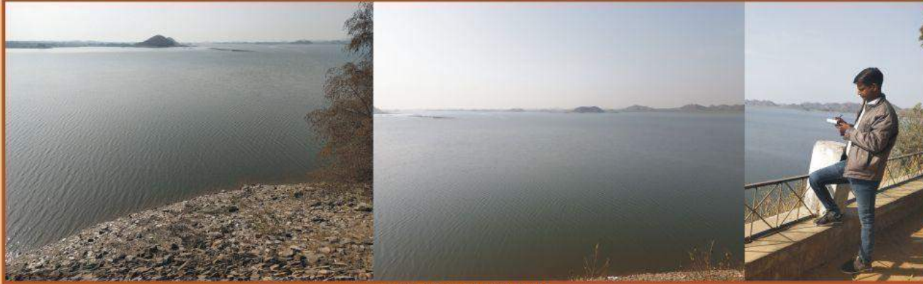
SURVEY OF GUDHA DAM
